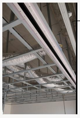
The installation take place between the spaces of the metal gypsum board by using threaded rods, according specification.
